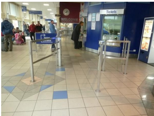
Figure 8: View towards the bus centre ticket desk with open barriers
